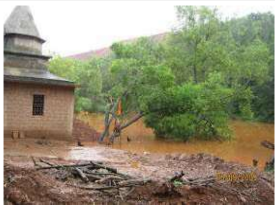
First lake location where traditional deiti Mhatrai temple was buried under the dempo mining rejection. New temple is under construction.
